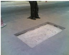
Figure (a): clean pothole and apply tack coat
